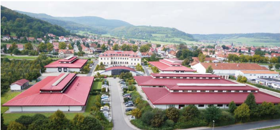
Plant Dermbach 36466 Dermbach, Thuringia total space: approx. 41,000 m 2
